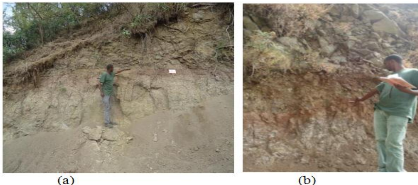
Figure-4.a) Contact between different flows of Ashange basalt: on the top part moderately weathered and fractured and the lower part is deeply weathered.
